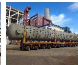
280 Tons of Steam Drum Water-land Transshipped From Zhangjiagang to Zhangzhou
